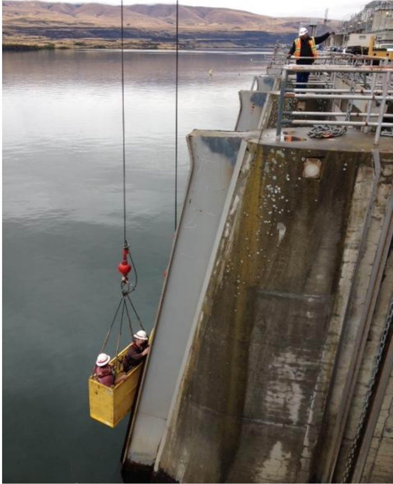
Derelict USGS I-beams on pier noses removed by project maintenance.
